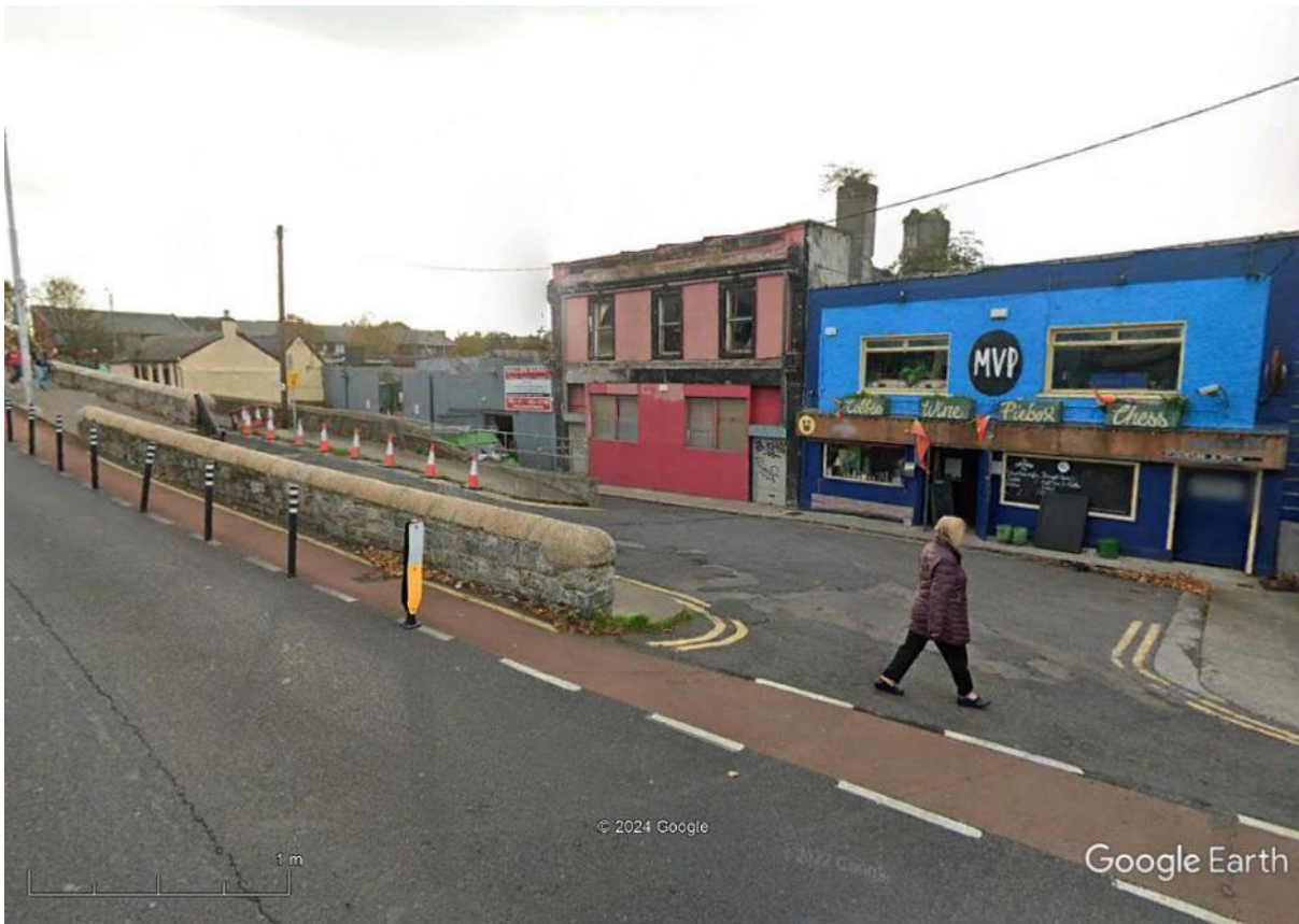
Figure 2-4-4: Street View of the Location from Clanbrassil Street Upper
