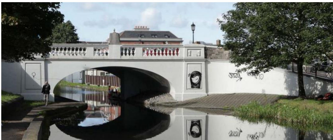
Figure 2-5-7: Existing View of Robert Emmet Bridge from the East
