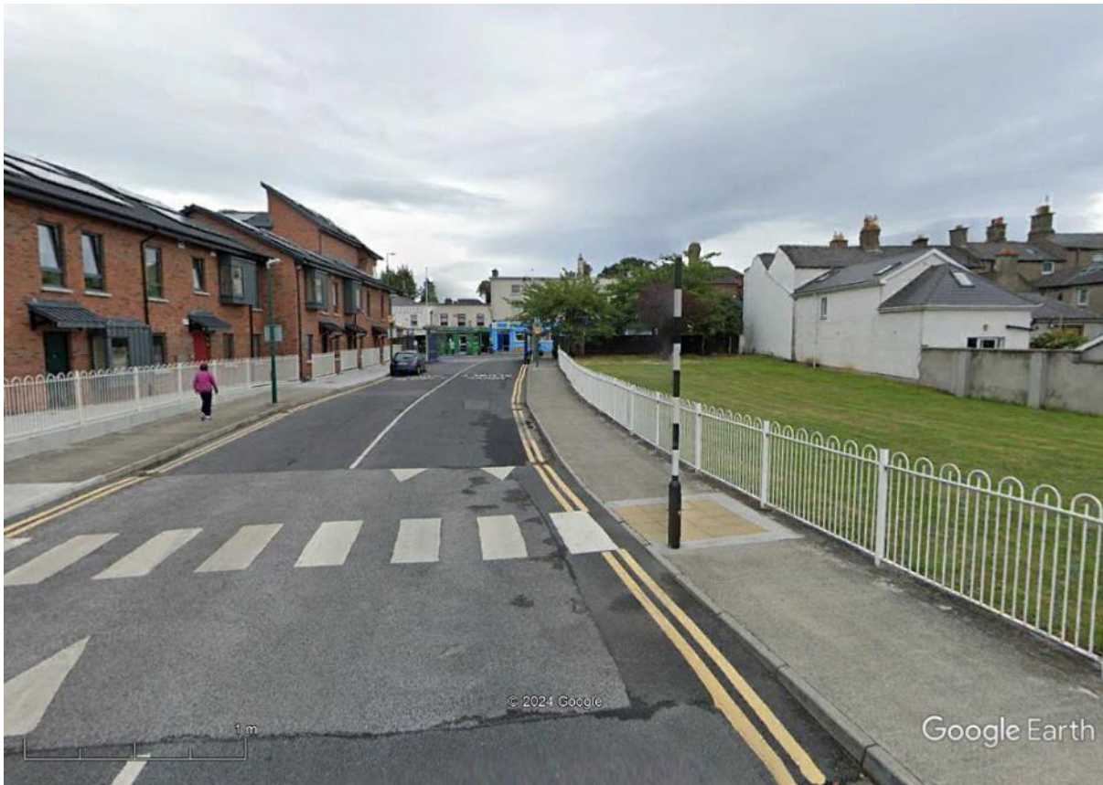
Figure 2-11-4: Street View of the Location looking east from within the Hospice
